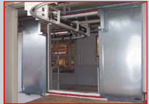
One of the first RGT conveyor system 1979
