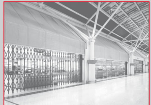
The first Fibershield E 240- Installed in Bolton , UK 1996
